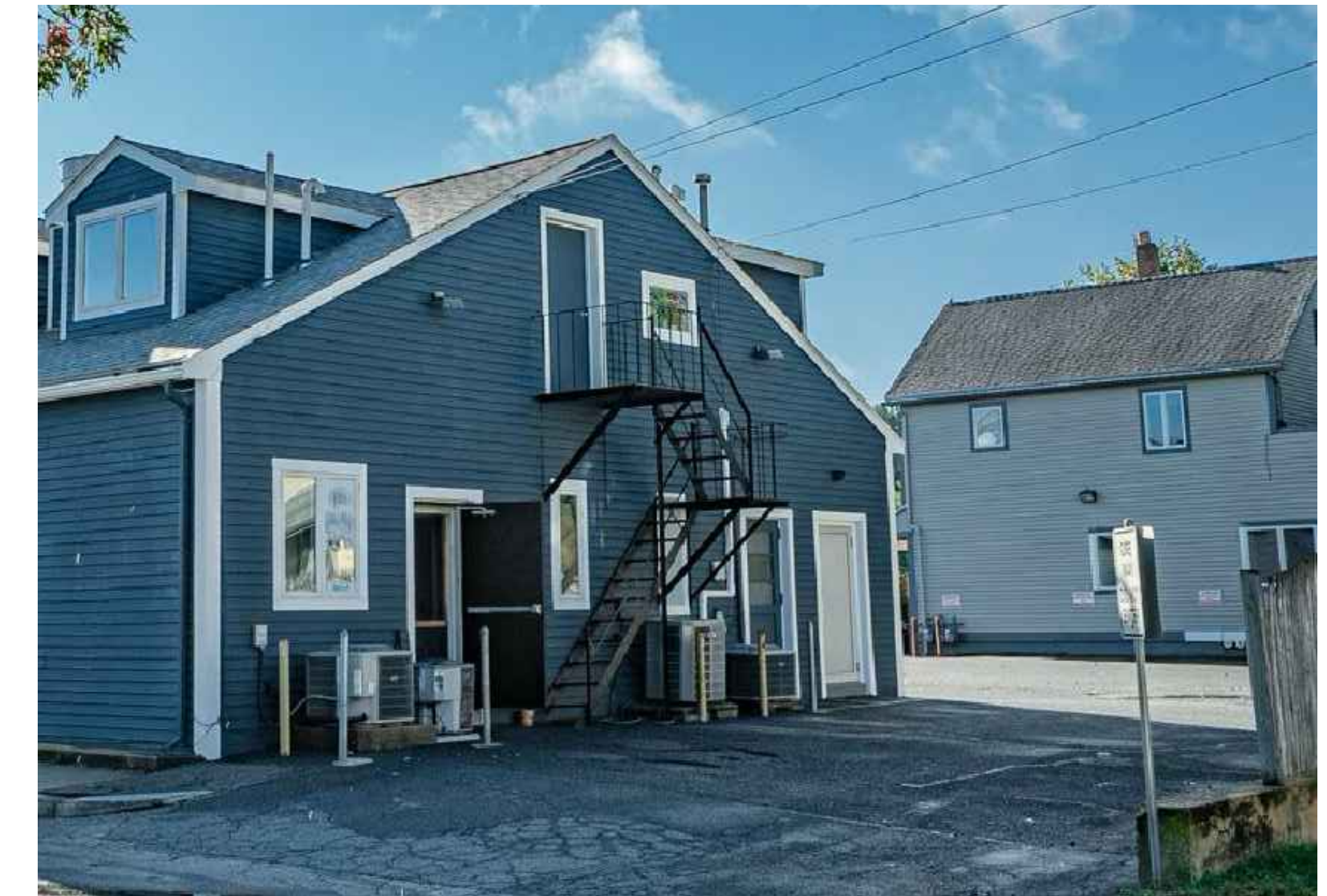
EXISTING REAR FACADE
