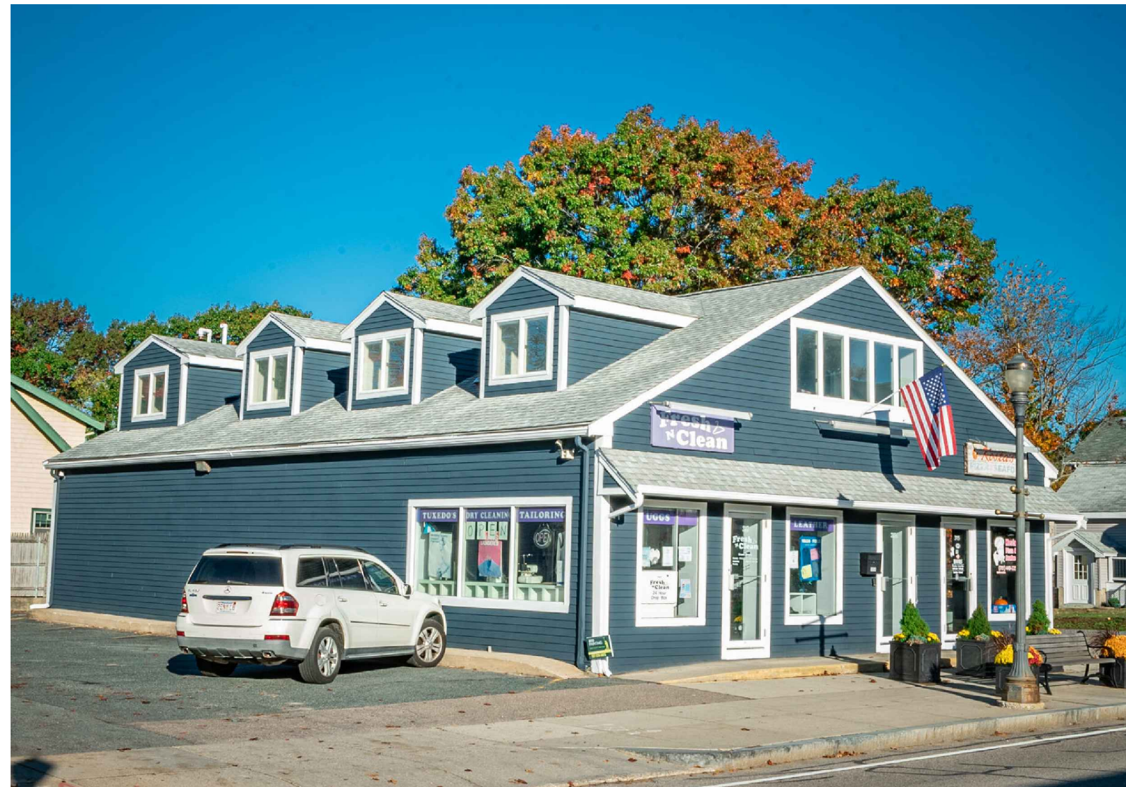
EXISTING LEFT SIDE FACADE PARKING LOT
