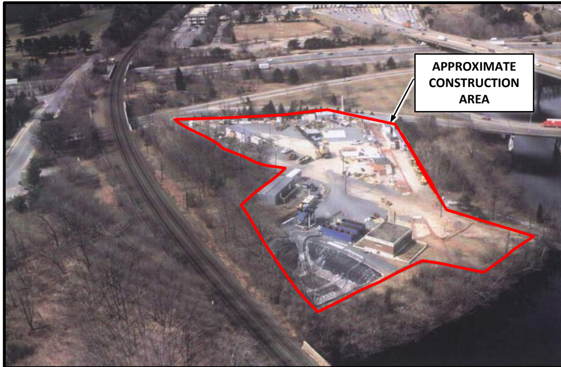
MWWST Shaft 5A – During Construction
