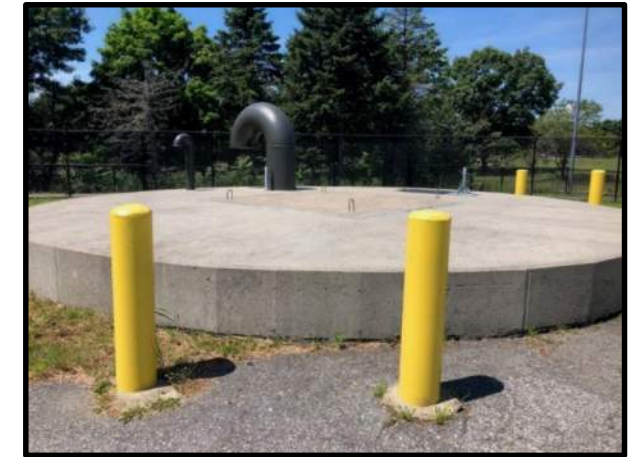
MWWST Shaft 5/5A, Weston
