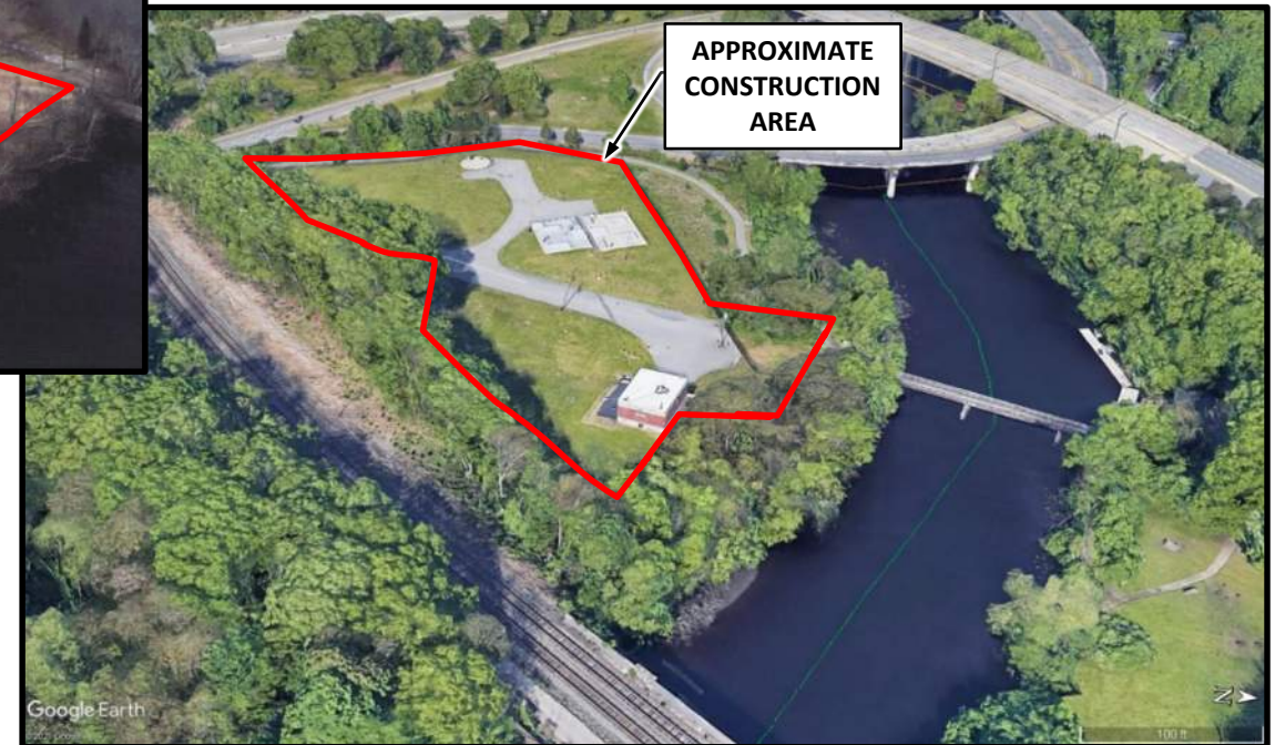
MWWST Shaft 5/5A – Post Construction
