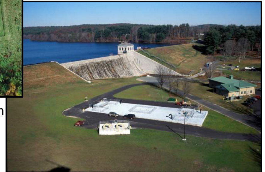
MWWST Shaft E, Southborough
