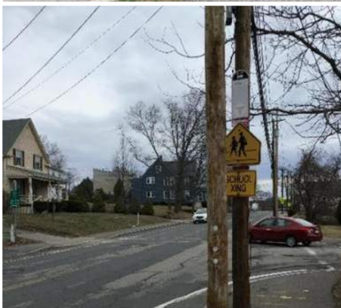
Non-MUTCD Compliant school crossing signage, also blocked by utility pole
