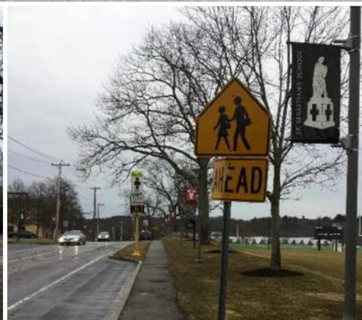
Non-MUTCD Compliant school crossing signage in poor condition on Greendale Avenue near St. Sebastian's School
