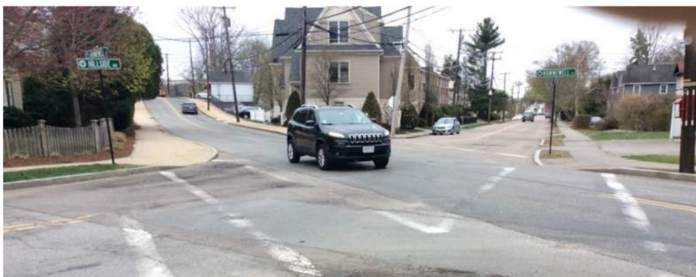
Faded pavement markings at Hunnewell/Hillside
