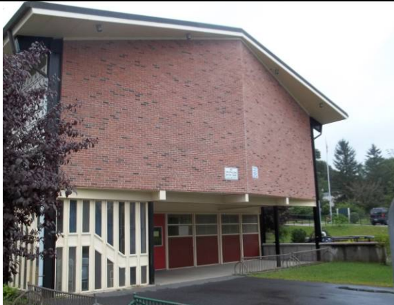
Photo #3: Side of building – facing west (lower level is cafeteria and upper level is gym)
