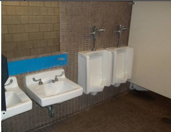
Photo #21: Restroom on ground level
