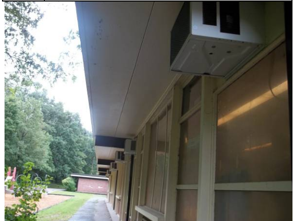
Photo #10: East side of building
