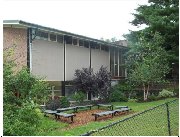
Photo #2: Front of building – facing south
