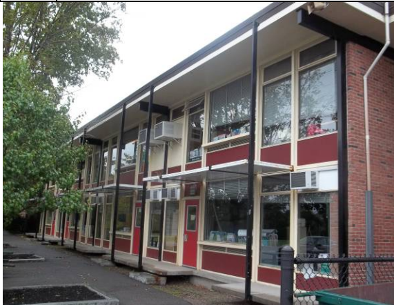
Photo #5: Side of building – facing west (classrooms on upper and lower levels)
