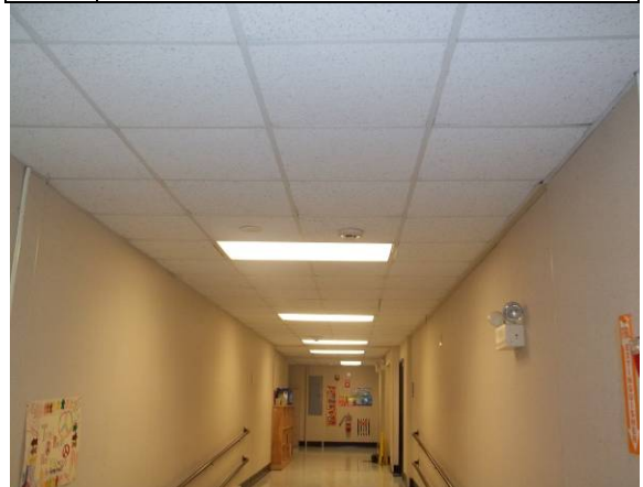
Photo #16: Modular section hallway – connects to ground floor main hallway
