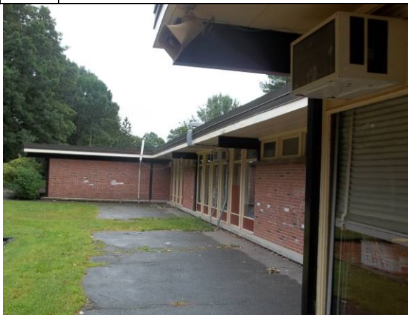
Photo #11: Additional view of east side of building
