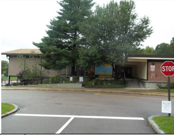
Photo #1: Front of building – facing south
