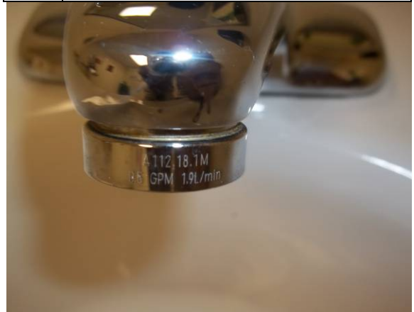
Photo #22: 0.5 GPM faucet
