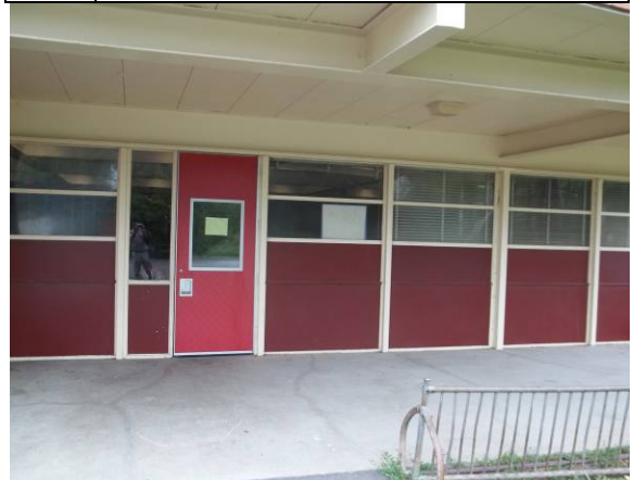
Photo #6: Entrance to cafeteria
