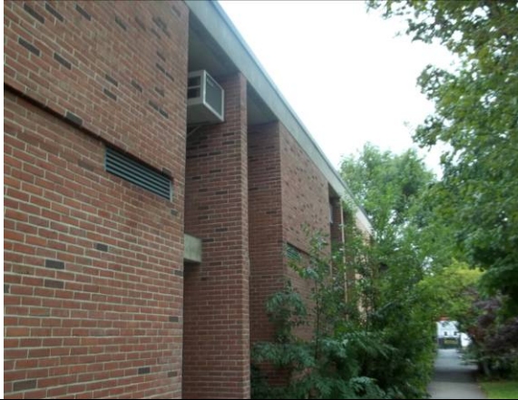
Photo #7: West side of building at the rear of the building
