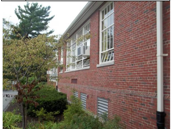
Photo #4: Closer view of front of building
