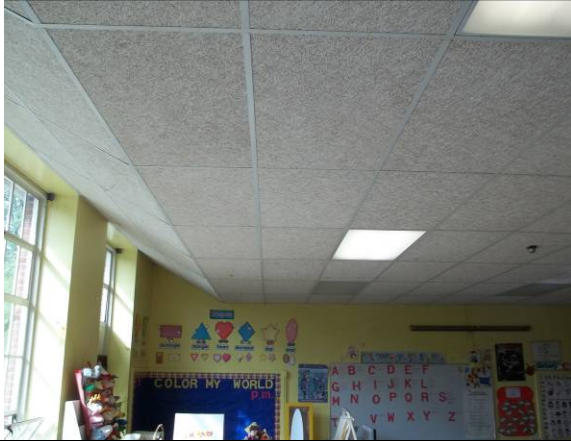
Photo #25: Several classrooms had lights adjacent to windows that provided enough light – recommend photo-sensors
