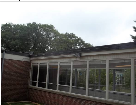
Photo #11: Hallway portion with sufficient outside light so that interior hallway lights should be on photo-sensors
