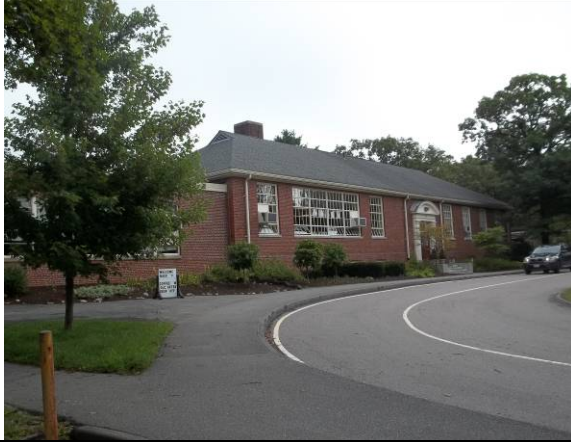
Photo #1: Front of building – facing south
