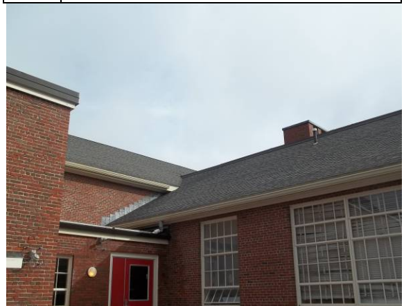
Photo #6: Roof – replaced in 2011
