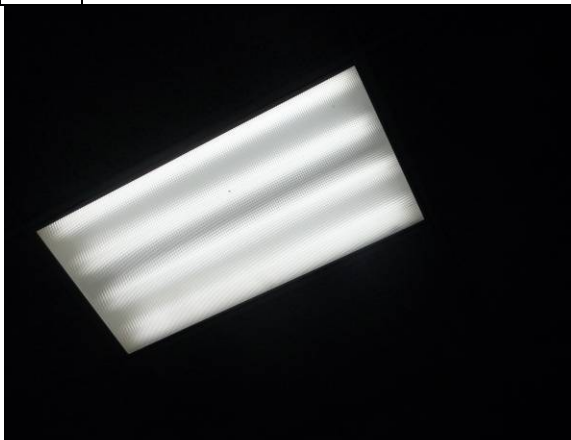
Photo #17: Hallway lighting – T8 lights
