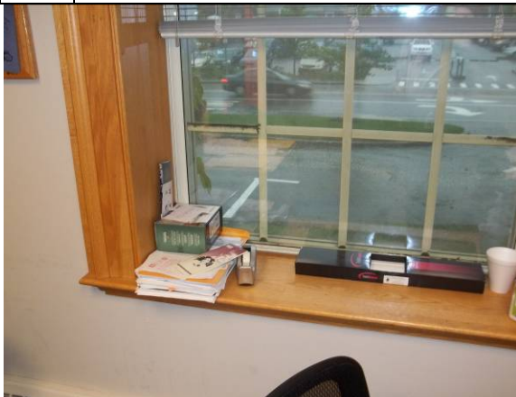
Photo #11: Aluminum framed double pane windows in office
