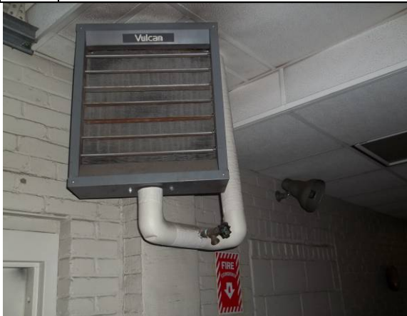
Photo #33: Hydronic unit heater – used in garages
