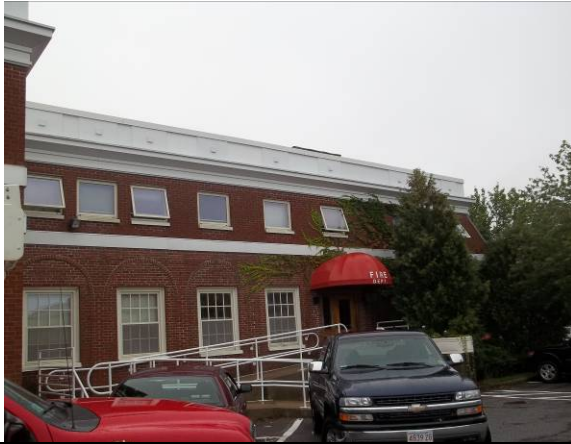
Photo #1: Fire department front entrance – facing north
