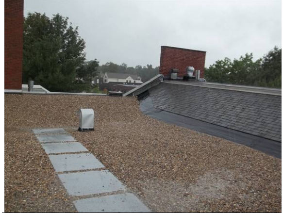
Photo #8: Roof of building
