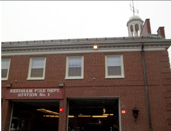
Photo #5: Fire department – facing west
