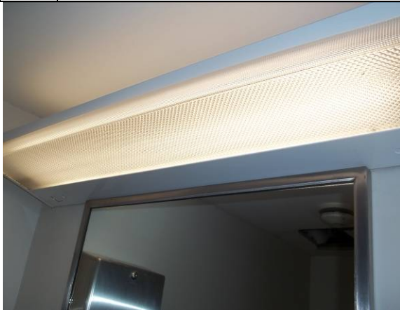
Photo #17: Restroom lighting
