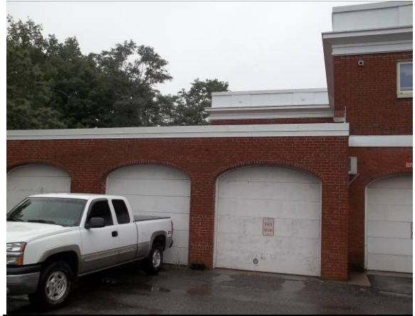
Photo #2: Fire department – garages facing north
