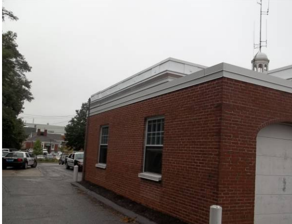
Photo #3: Side of building – facing east
