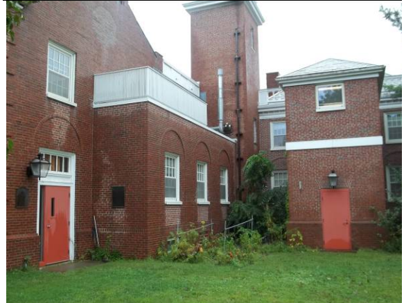
Photo #6: Building facing west
