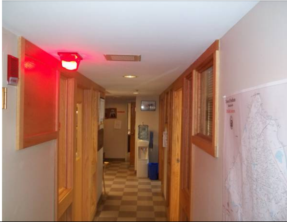
Photo #25: Fire department hallway
