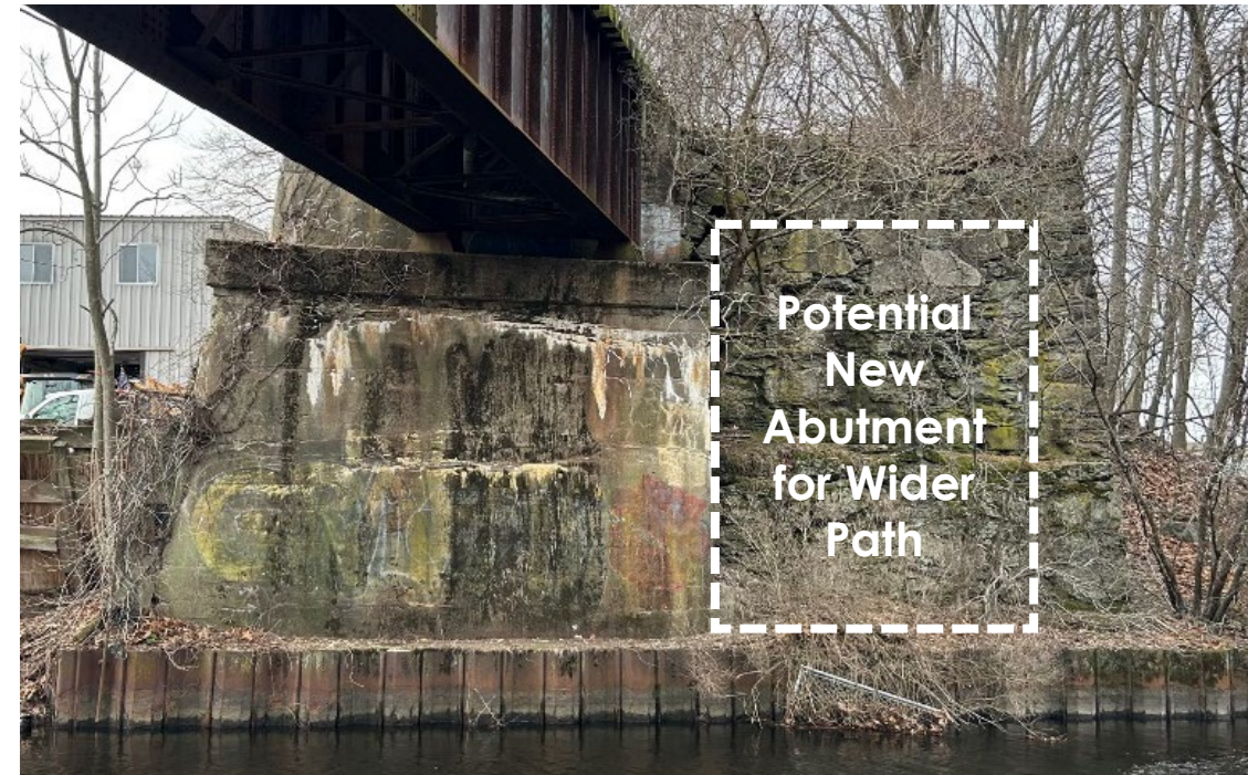
Existing South Substructure
